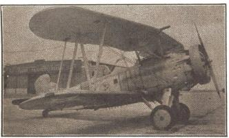
PRESENTING Curtiss' new Helldiver FSC-4 now being used for dive bombing by several Navy squadrons. This "shot" is interesting, since it shows the upper-wing gun and the special bomb racks fitted beneath the wing.
