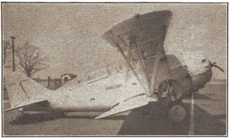
THE Navy is going in strong for the Grummans! This is the new XSF-2 two-place shipboard fighter. It mounts a Twin-Wasp, which gives the craft considerable more speed than the original model which employed a 710-hp. "Cyclone" and had a top of 197 mp.h.
