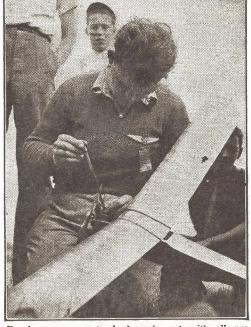
Eye-droppers are standard equipment with all gas jobbers. Above we see Ira Hassad, of California, feeding his tiny ½-inch bore engine with one. Ira designed and built this unusually small plant. The model in which it is mounted carries 300 square inches of wing surface.
